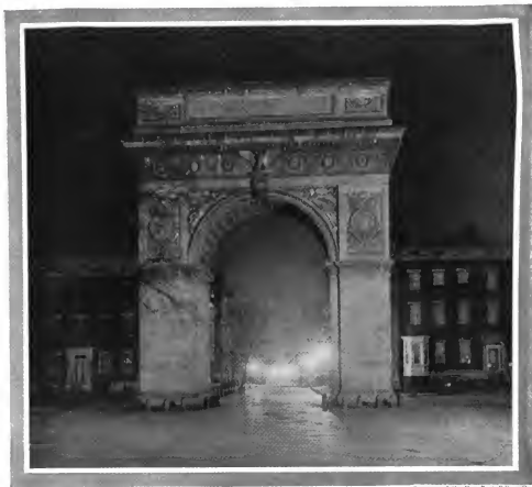
Courtesy of the New York Edison Co.
